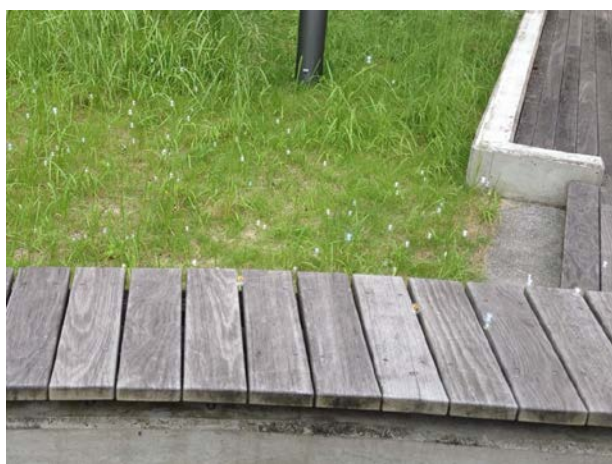
Figure 21. No. 1 soap bubbles outdoors. The soap bubbles were stable on grass and a wooden deck
